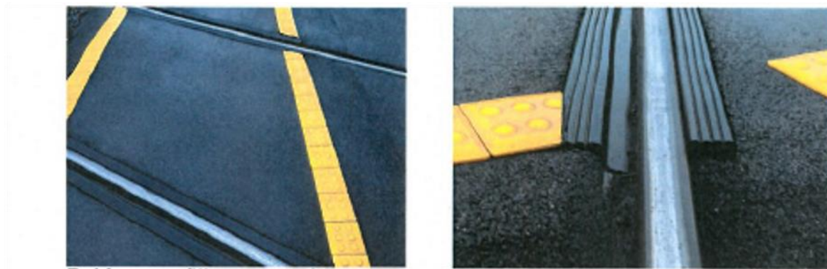
Rubber gap fillers at the Charman Road Level Crossing, Cheltenham
